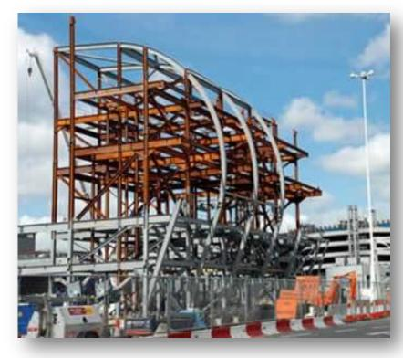
The curved steel beams were 27m long and each one weights about 14.5 tonnes. The Terminal 2 building first phase contained six of these huge beams.
