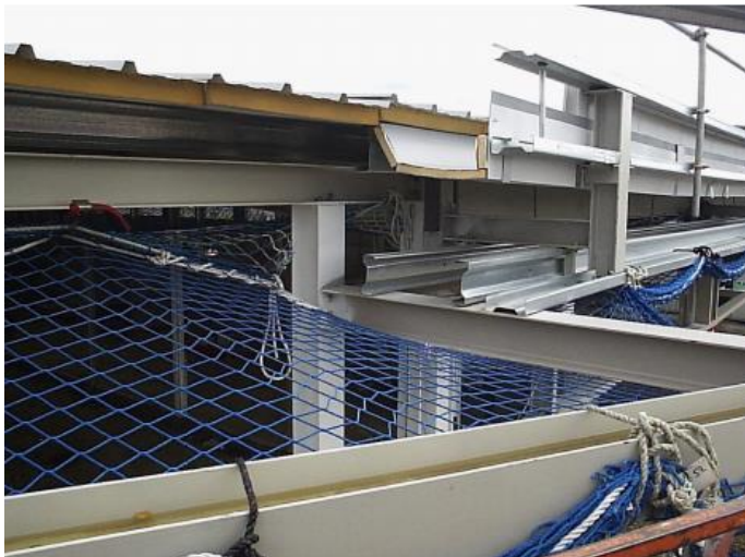
GUTTER DETAIL - INTERNAL - AUGUST 2007
