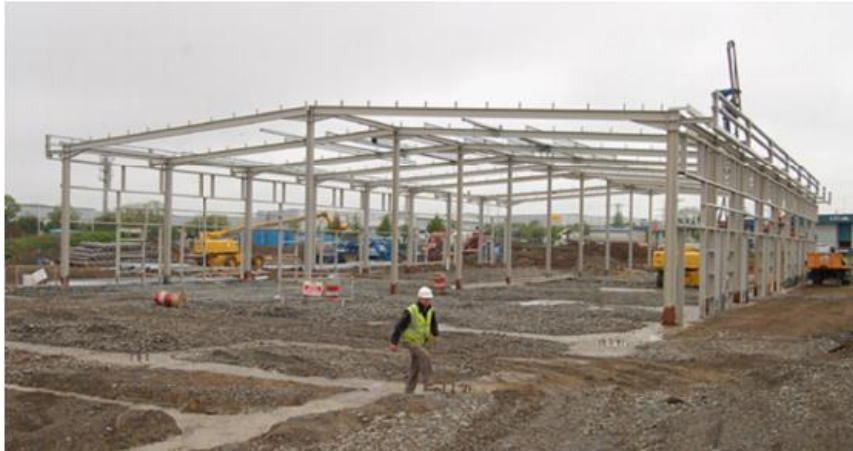
STEEL FRAME - MAY 2007
