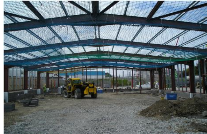
STEEL FRAME - JUNE 2007
