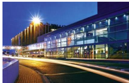
Figure 1: Dublin Airport (Terminal 1)
