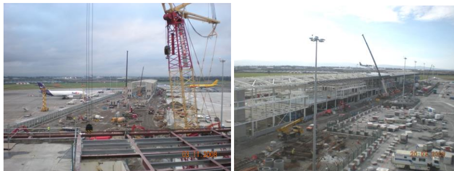
Figure 4: Pier E Construction Photos (November '08 to February '09)
