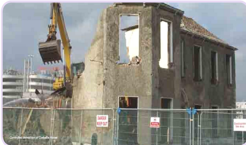
Figure 2: Historical Corballis House being taken down.
